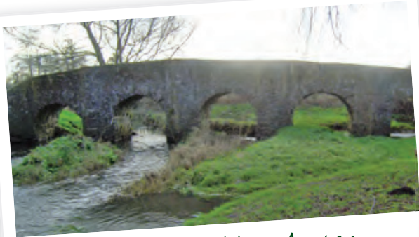
Packhorse Bridge, Anstey
